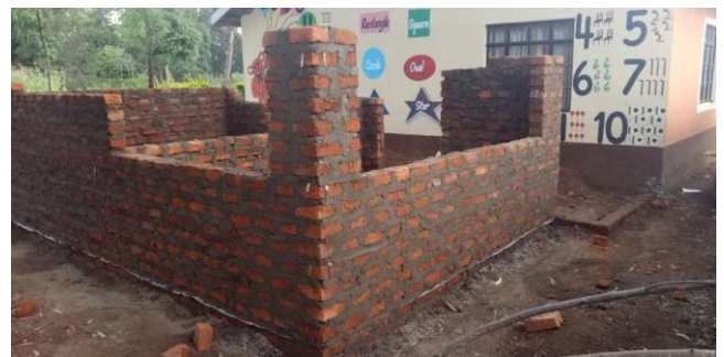
ECD Kitchen under construction
